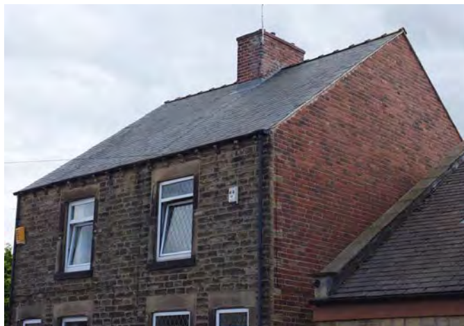
Photo 12 – Historic property with stone front elevation and brick elevations to side
