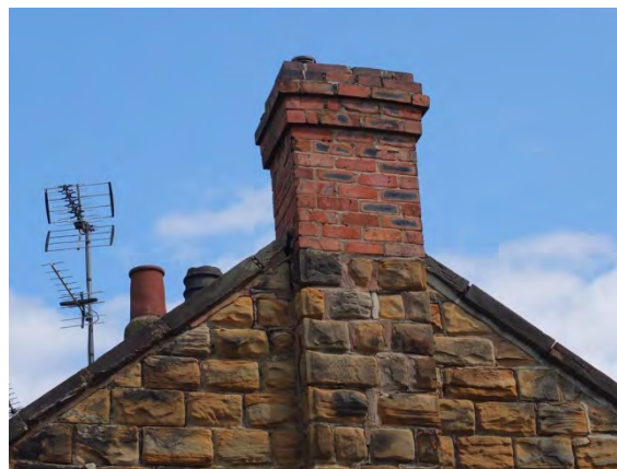
Photo 2 – replaced brick flue with over-sailing courses
