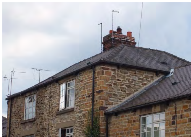
Photo 5 – hipped Welsh slate roof (Station Row)
