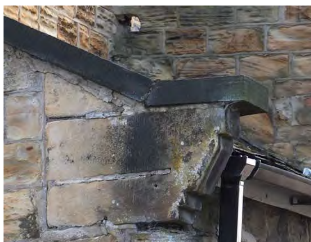
Photo 8 – Kneeling stone at the edge of the gable, supporting the verge coping
