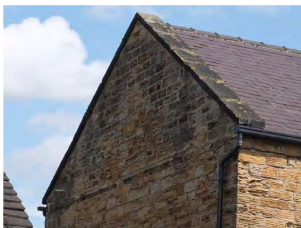
Photo 6 – Welsh slate gable roof with verge coping
