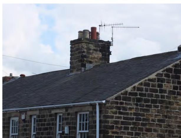
Photo 7 – Welsh slate gable roof with mortar fillet finish
