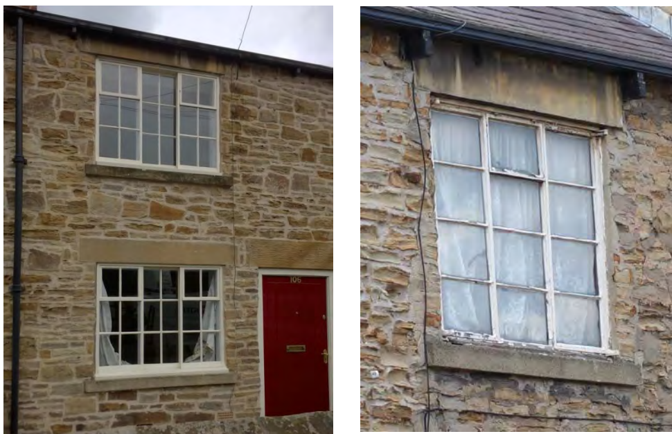
Photos 26 and 27 – Yorkshire sash replacement windows (Reform Row) and metal casement (Station Row)
